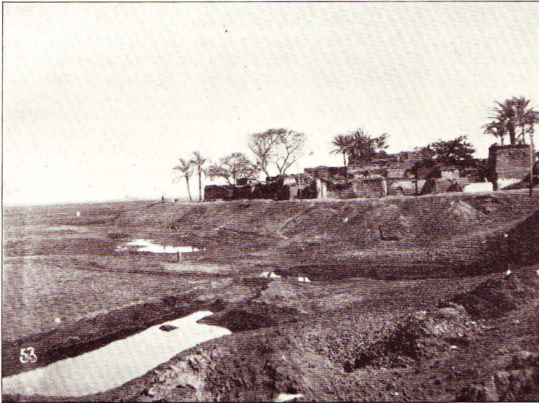
A VILLAGE BUILT ABOVE HIGH NILE LEVEL.
